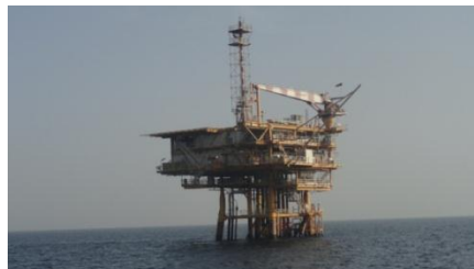
Central Monitoring Station (top) & Oil Platform (bottom)
