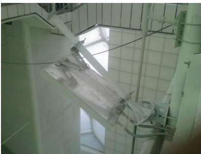
Fig 8 & 9: Narrow beam antennas installed along runway
